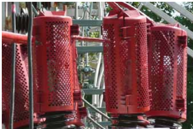
BCAC-IC Installed on Bushings
