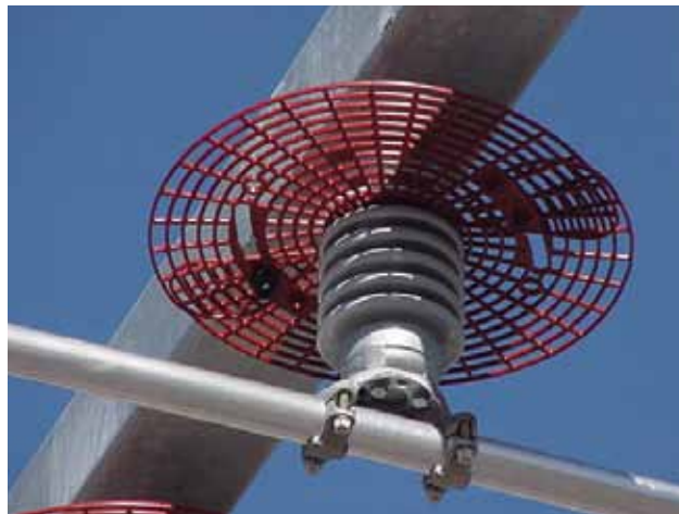
BISG-60/115-02 installed on bus support insulator
